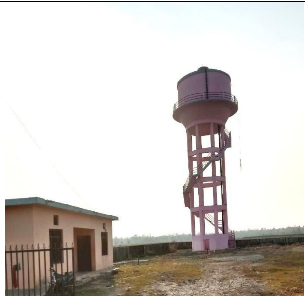
2. Existing structure at the Matgaura Water Supply Project, OHT premises
