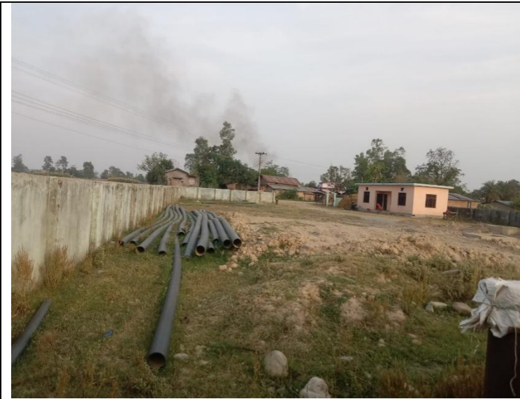
1. Existing office building of Matgaura WSP
