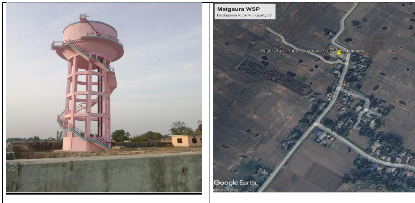
Figure 222: Location of proposed land for Matgaura Water Supply Project and google Map
